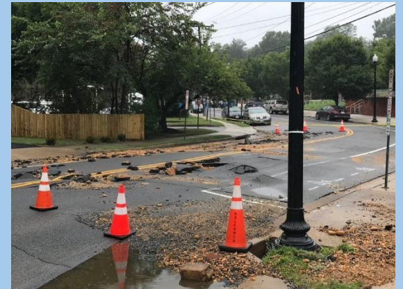
Surface damage on 18 th Street North following July 2019 floods in Arlington. Photo credit Arlington DES.
